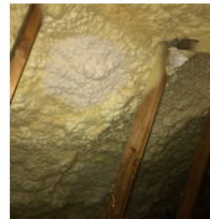
Figure 1 and 2 A portion of the foam was removed, the monitor was attached to the bottom of the roof decking, covered with plastic and the spray foam was reapplied to
